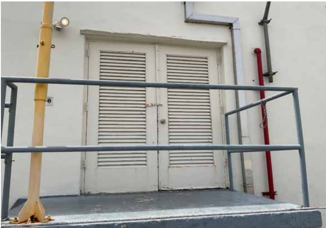
Doors - Bldg C Pump Room
