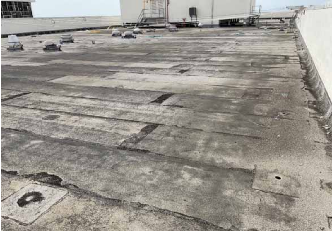
Bldg C Roof
