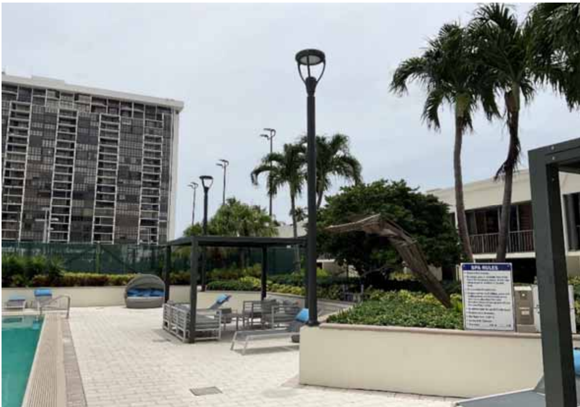
Light Pole & Fixture - Pool Deck
