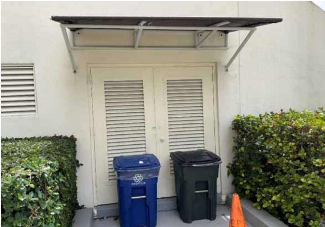
Doors - Townhouse Mechanical Room
