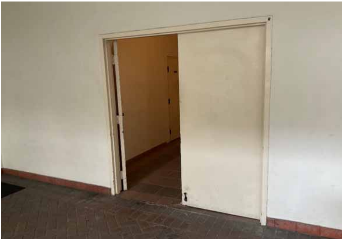
Doors - Bldg D Storage Area
