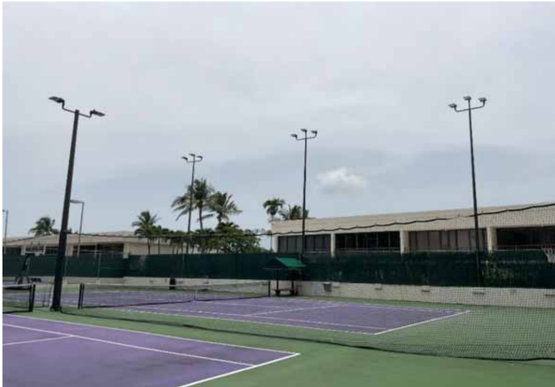
Tennis Court Light Pole & Fixture
