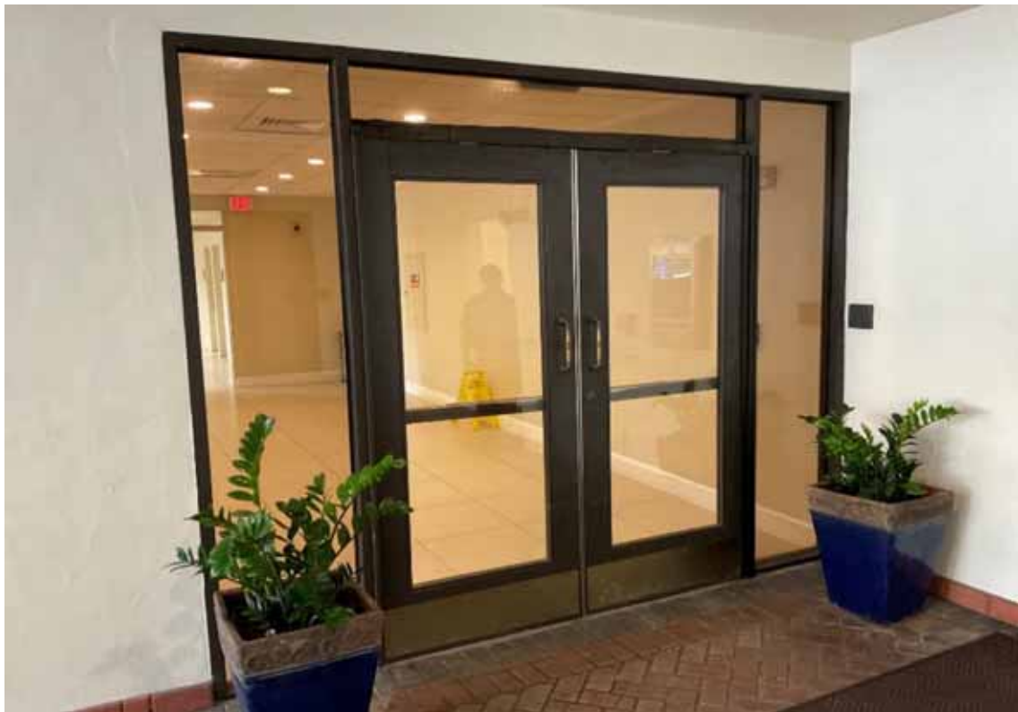
Windows & Doors - Bldg D 2nd Floor Entrance
