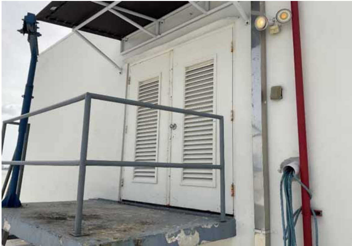
Doors - Bldg D Pump Room
