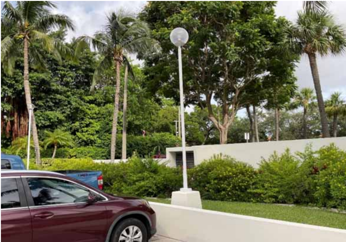
Light Pole & Fixture - Parking Deck
