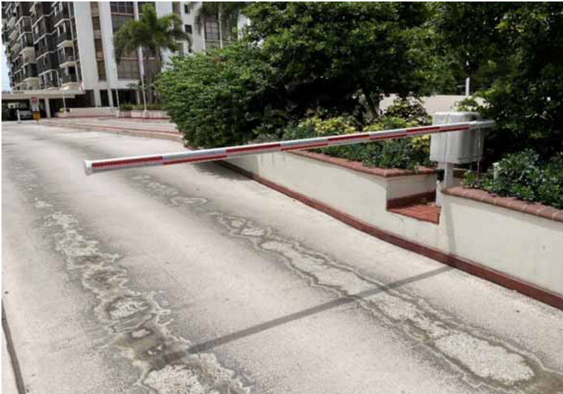
Resident Entry Barrier Gate
