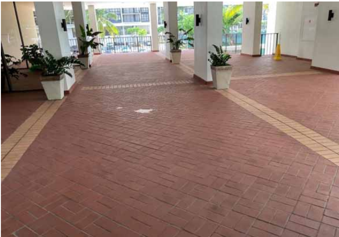
Bldg C Paver Walkway
