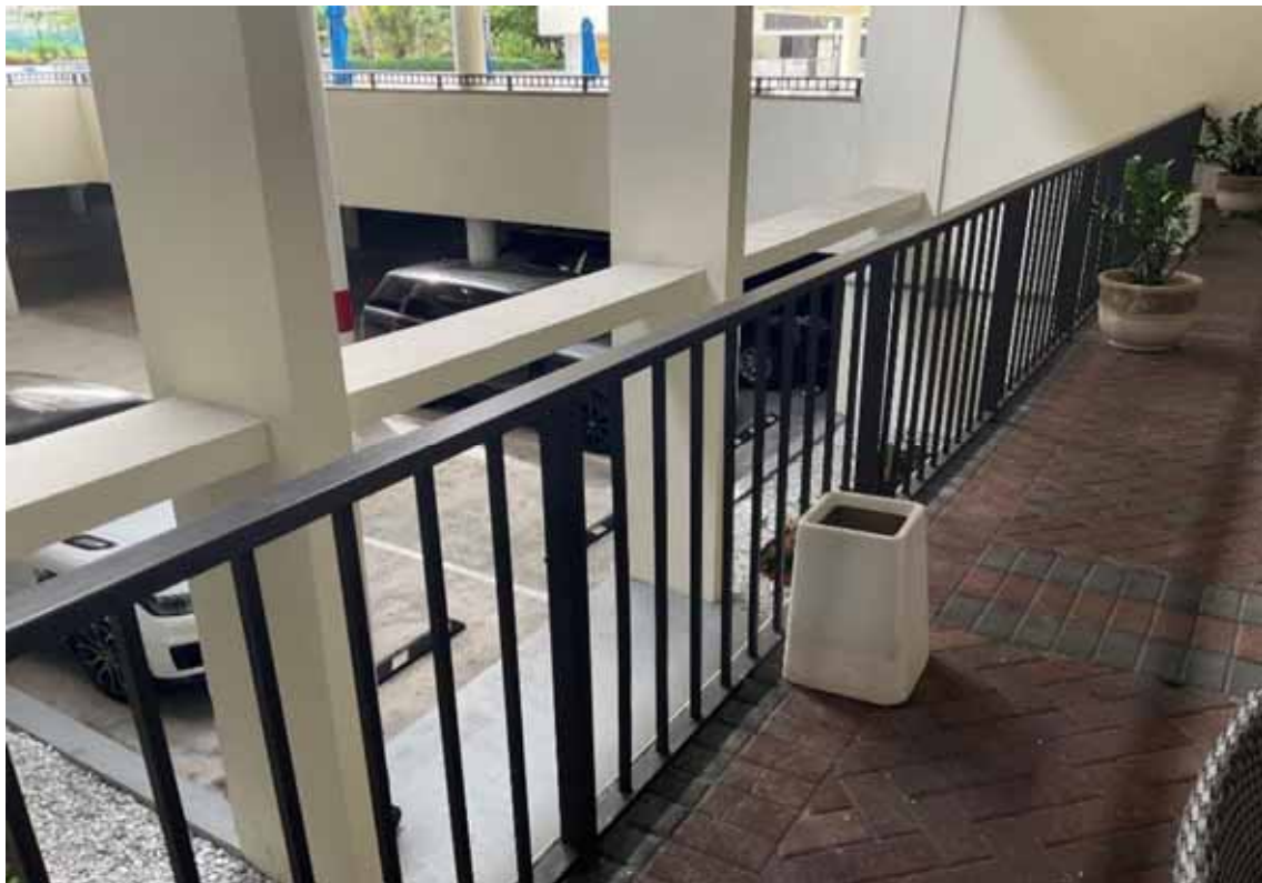
Bldg D Walkway Railing
