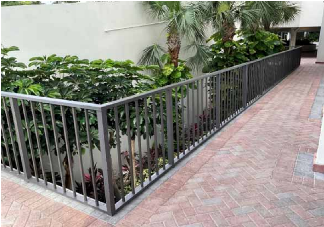
Bldg D Walkway Railing
