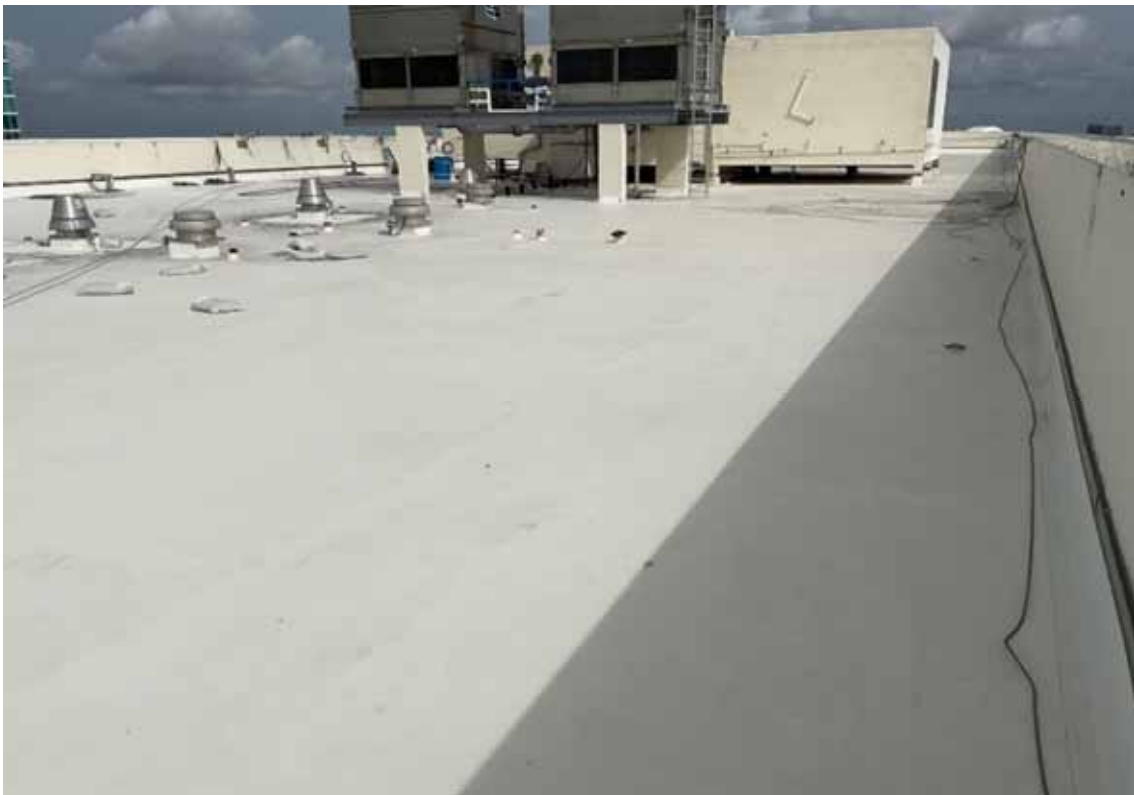
Bldg D Roof
