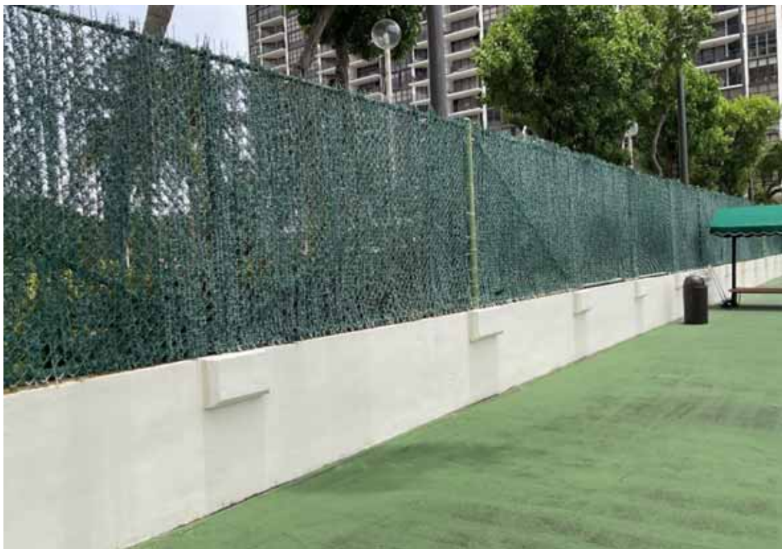
Tennis Court Fence
