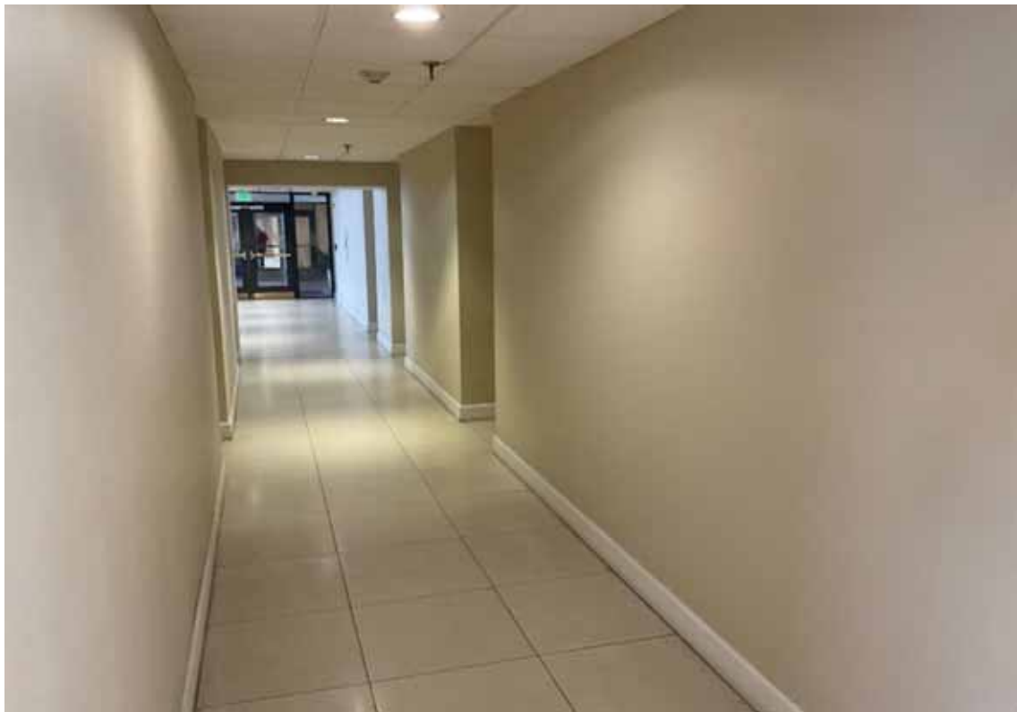
Bldg C Hallway - 2nd Floor
