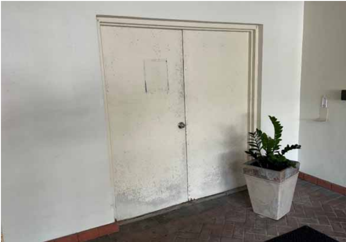
Doors - Bldg C Storage
