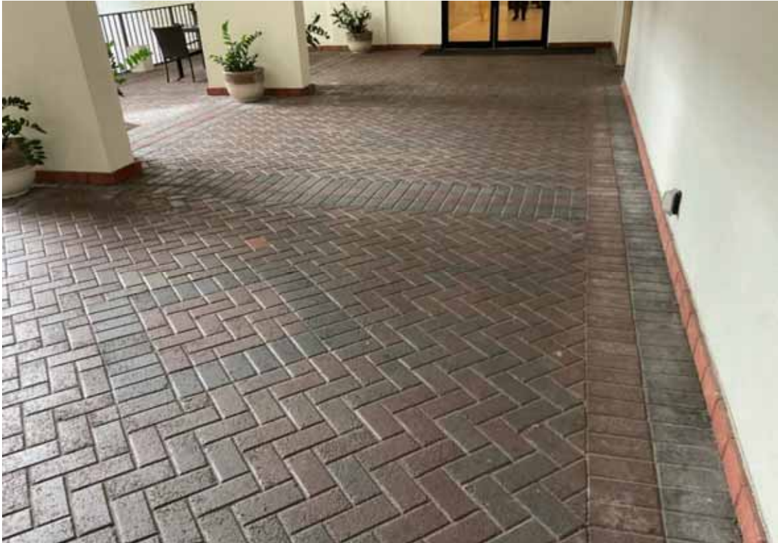
Bldg D Paver Walkway
