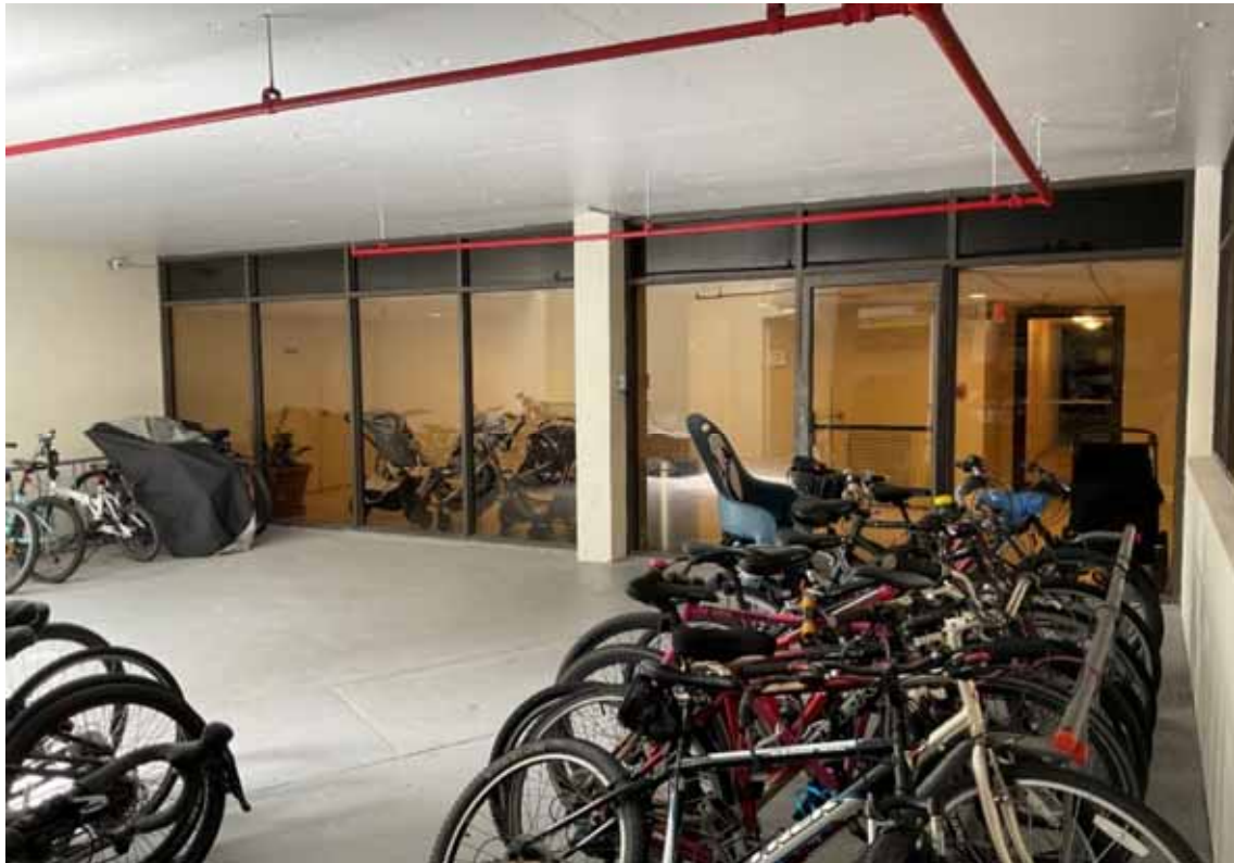
Windows - Bldg D Garage Lobby
