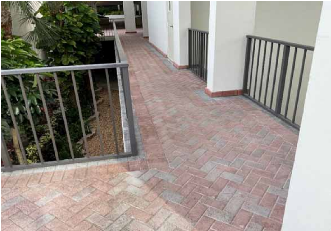
Bldg D Paver Walkway
