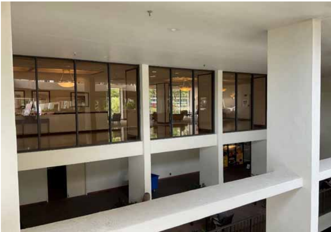
Windows - Bldg D Lobby
