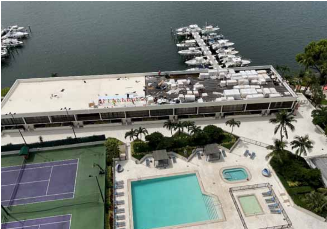
Townhouse Bldg Roof
