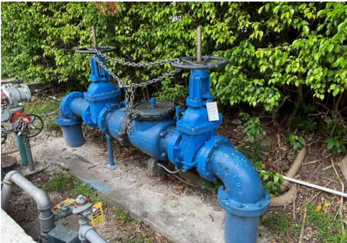
Backflow Preventer - Domestic Water
