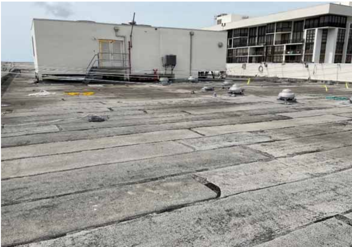
Bldg C Roof
