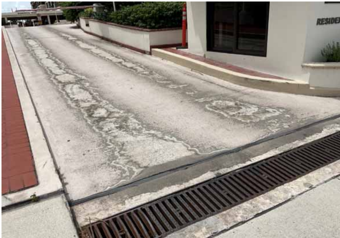
Resident Entry Ramp
