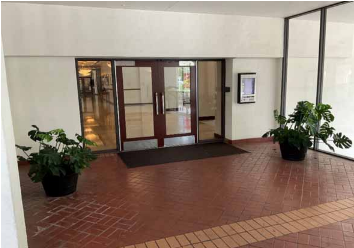
Windows & Doors - Bldg D Lobby Entrance
