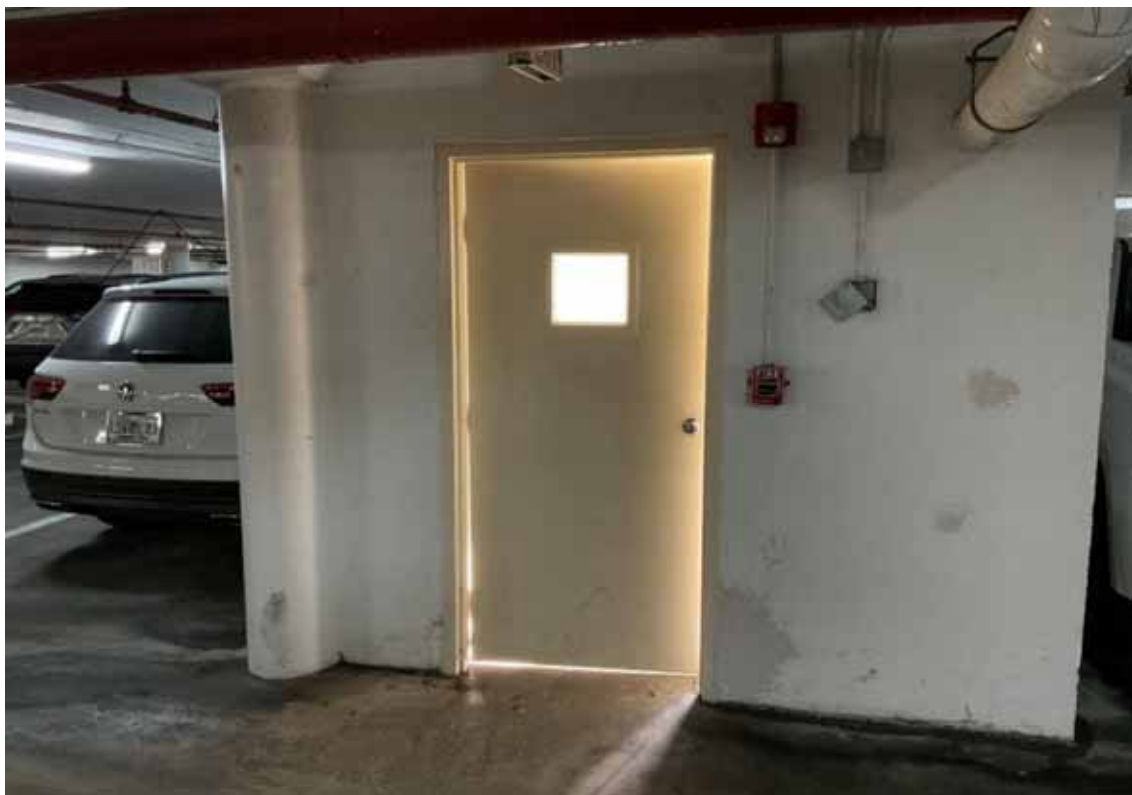
Door - Parking Garage Stairway
