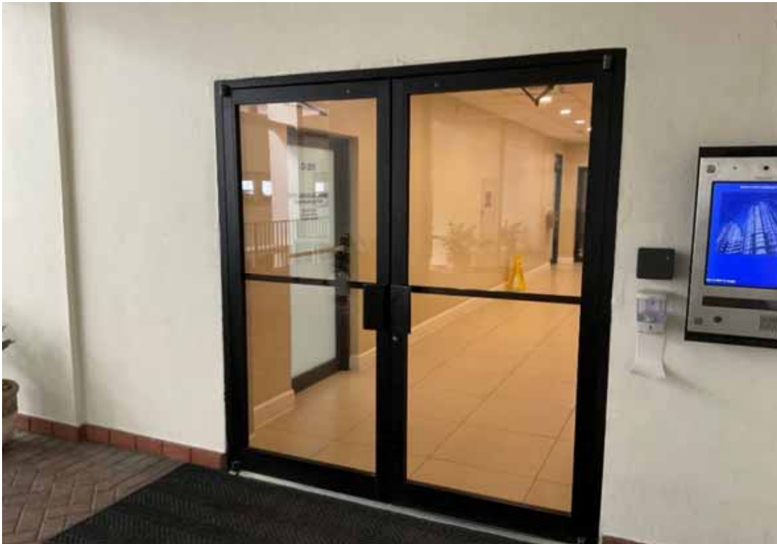
Doors - Bldg D 2nd Floor
