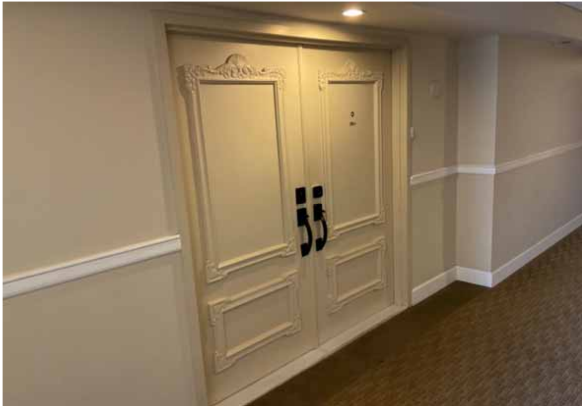
Bldg C Unit Doors - Penthouse Floor
