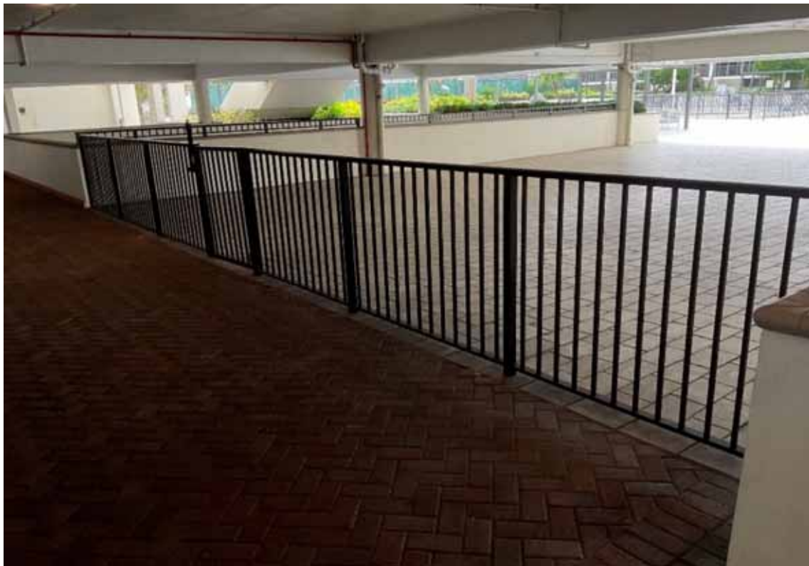
Pool Area Fence & Gate
