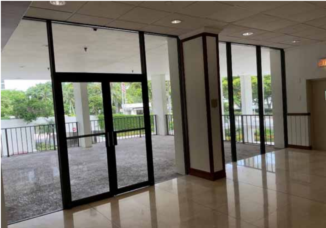
Windows & Doors - Bldg C Lobby Patio
