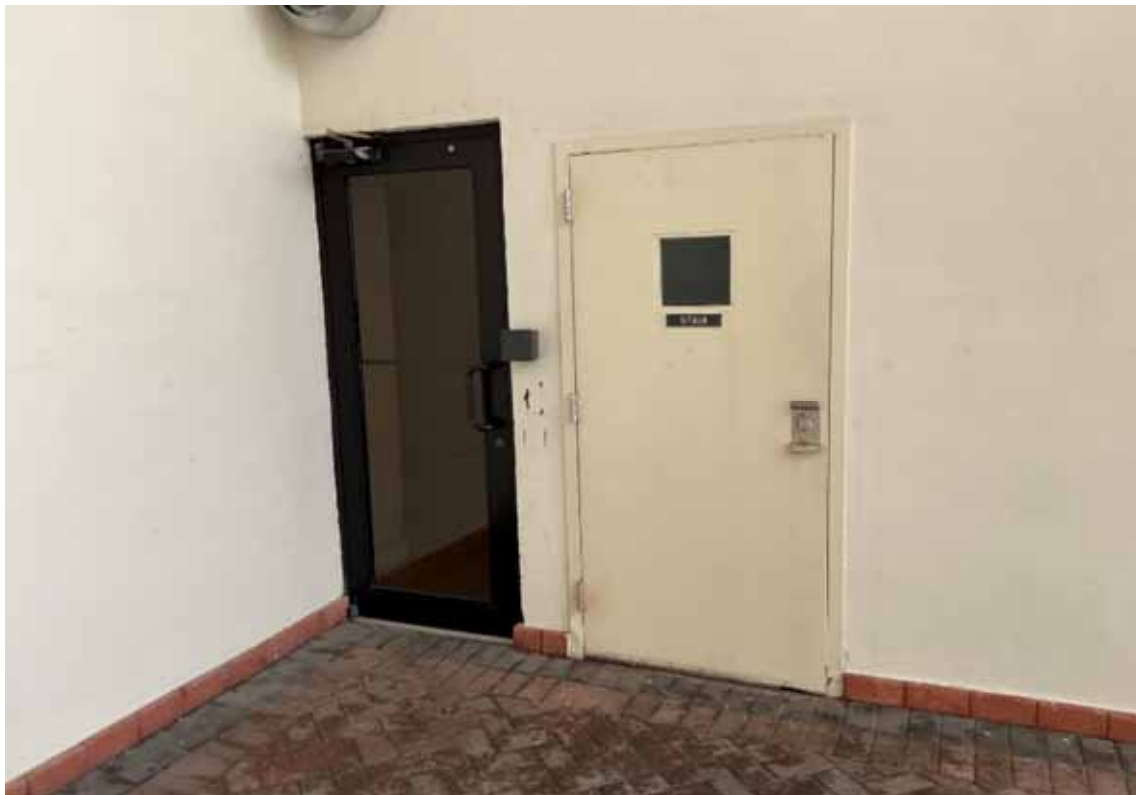
Doors - Bldg C 2nd Floor
