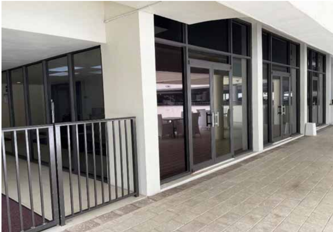
Windows & Doors - Bldg C 2nd Floor
