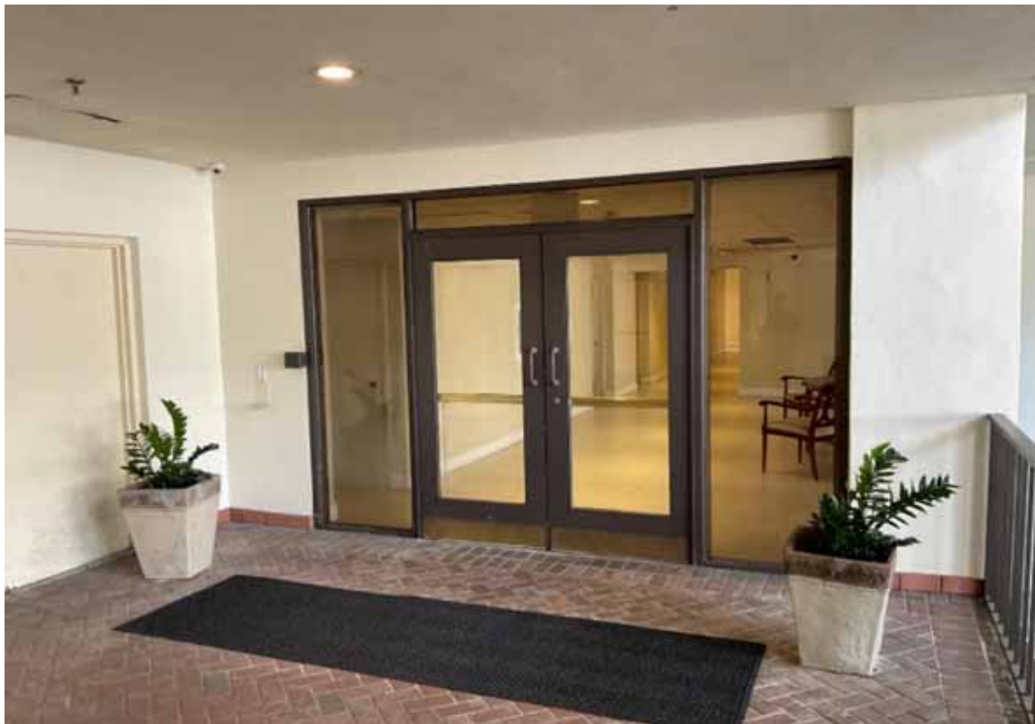
Windows & Doors - Bldg C 2nd Floor Entrance
