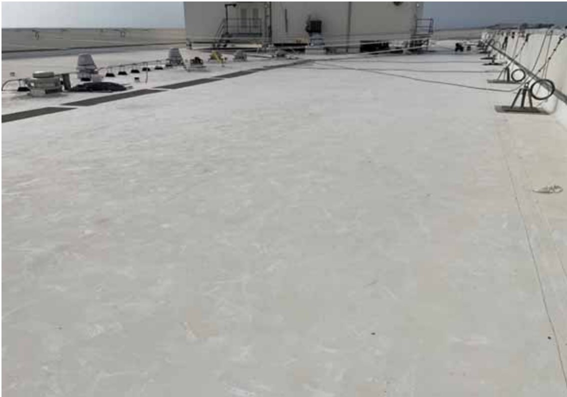
Bldg D Roof
