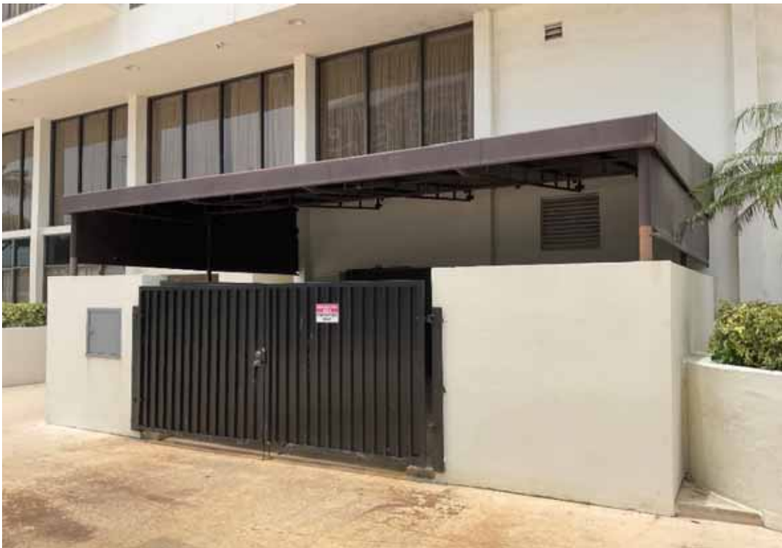
Bldg C Trash Room Awning
