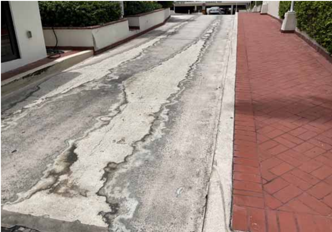
Visitor Entry Ramp
