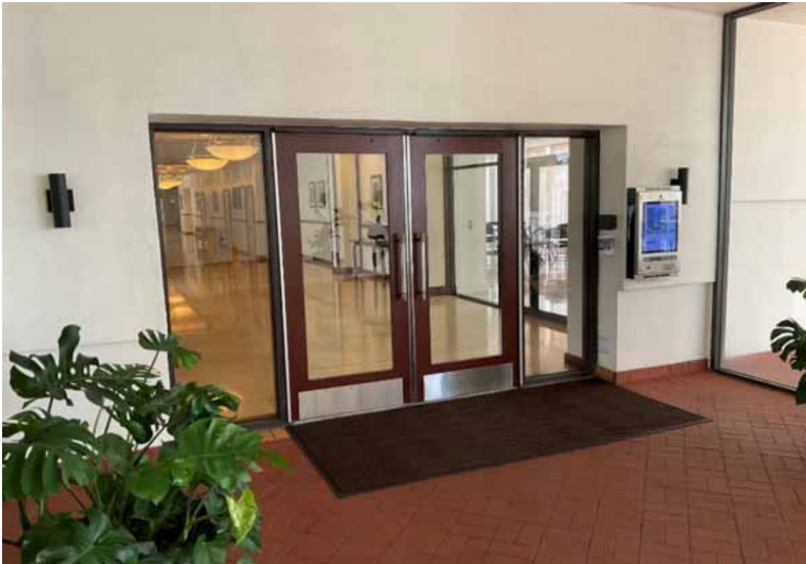
Windows & Doors - Bldg C Lobby Entrance
