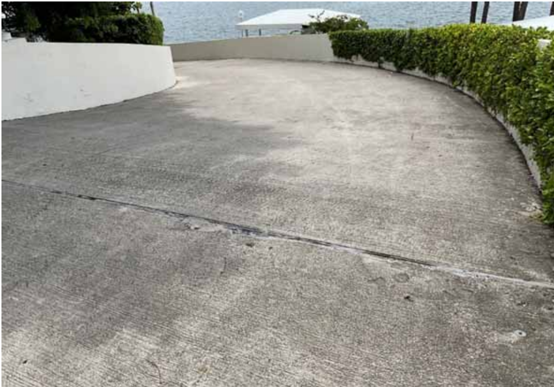
Marina Access Ramp
