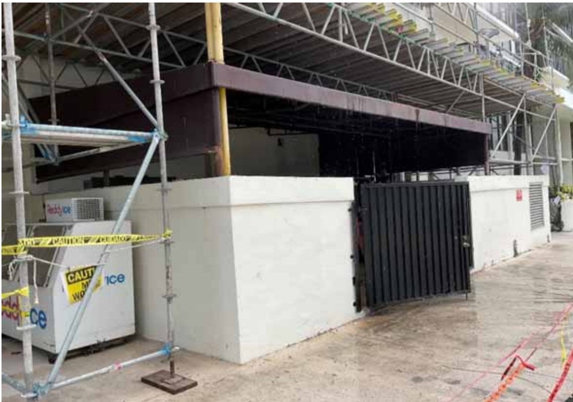
Bldg D Trash Room Awning
